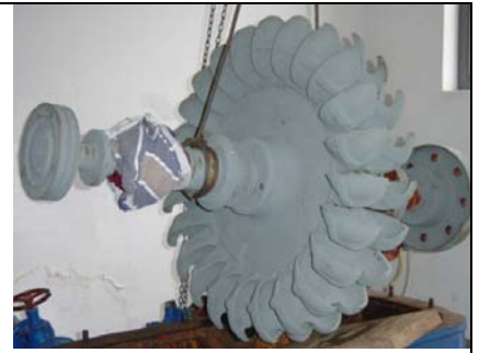
THE RECONDITIONED PELTON WHEEL BEING LOWERED INTO THE CASING. SEPTEMBER 2003
